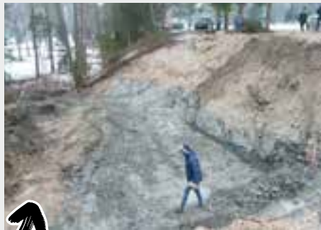
Visit the construction site
