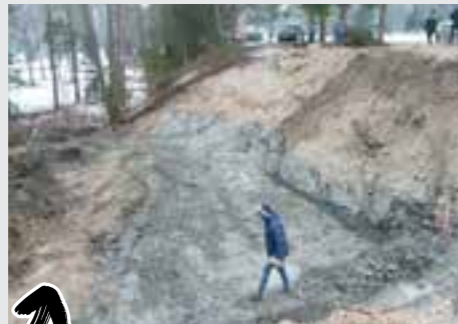
Visit the construction site
