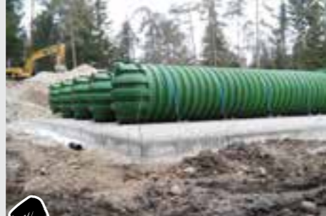
Installation of products and hand over the required technical documentation
